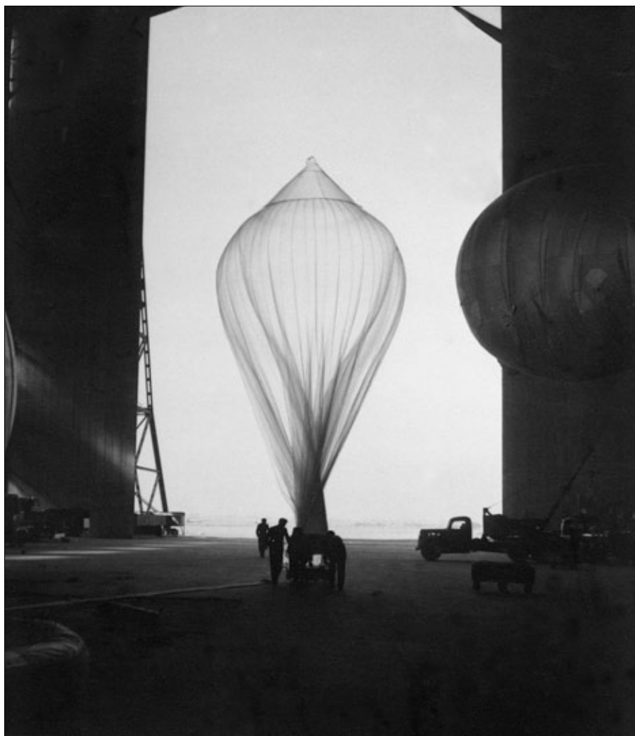
Figure 2.6. Bristol University balloon, 1953. The inflated balloon is being wheeled out to the tarmac for launch. Inflation took place inside a 120-foot-tall hangar, originally used for airships. Hydrogen was available through a 10-inch spigot on the hangar floor. (Photograph: by the author.)
